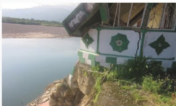
Collapsed of wall due to flood caused by heavy rainfall at Balat Village.
