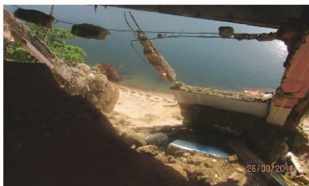
Collapsed of wall due to flood caused by heavy rainfall at Balat Village.
